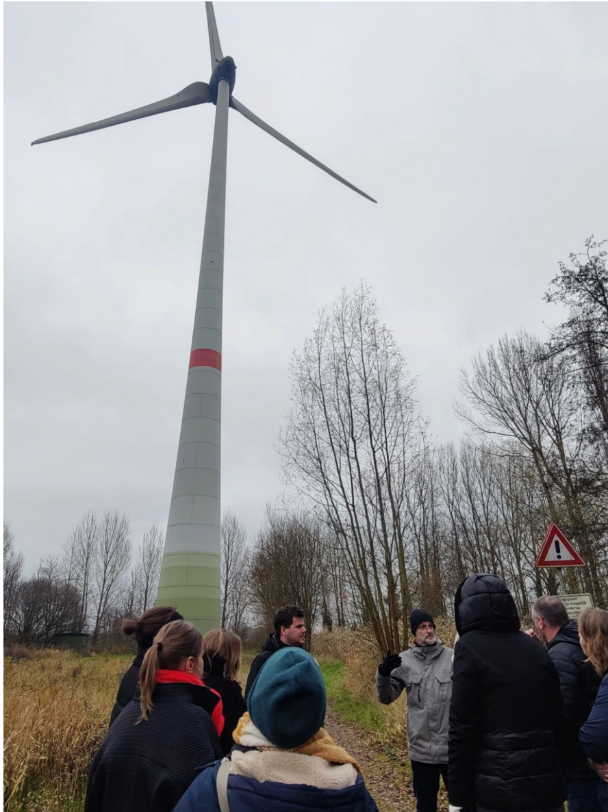
Figure 3 – Site visit in one of Eeklo's wind turbines during the national capacity building workshop.
